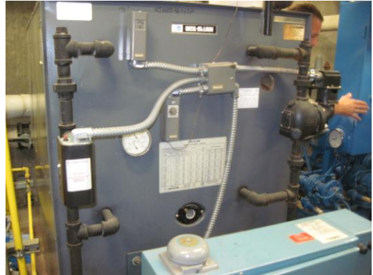
Existing DHW Heaters
